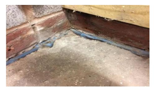
4) Due to Concealed Plumbing and Conduit pipe Leakage of Loose Joint.
